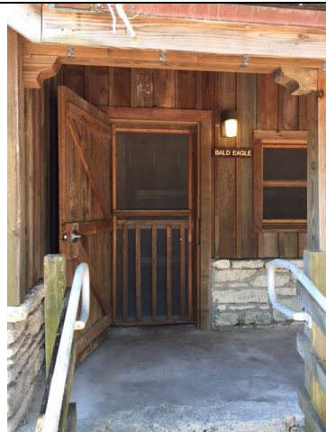
One of the cabins at Camp Greynolds
